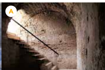
▲ Staircase going down to the inside the cistern from the courtyard
