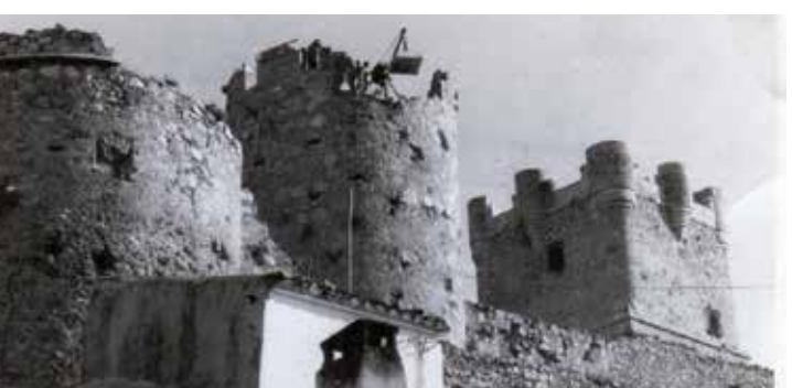
▲ Restoration works in 1960
